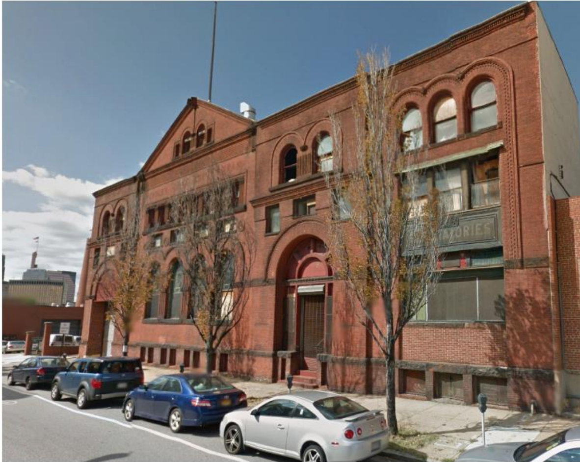
Image 11: Main (South) Facade, Hendler Building, 2017
