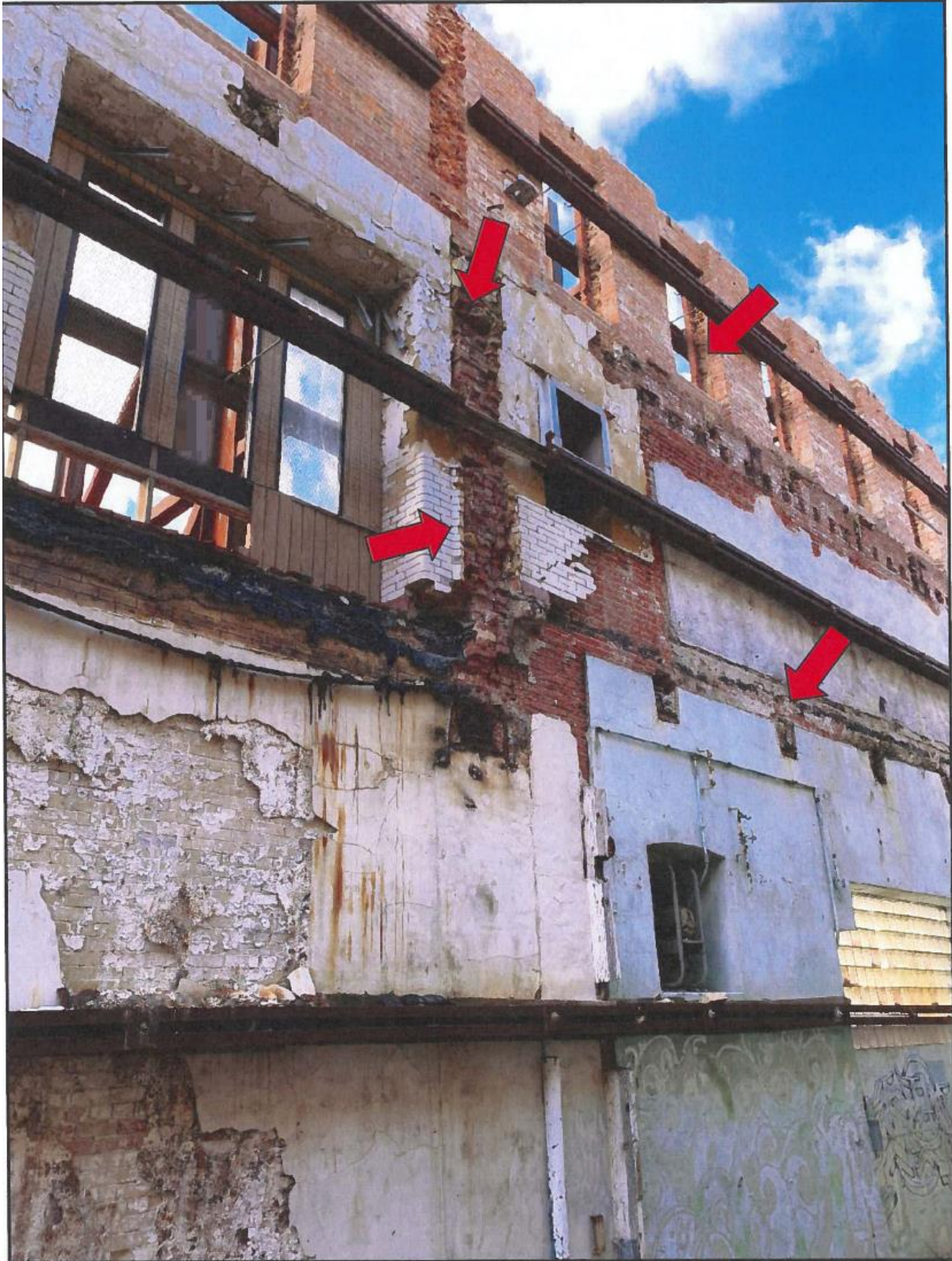
Image 23: Existing Conditions, Hendler Building, 2023
