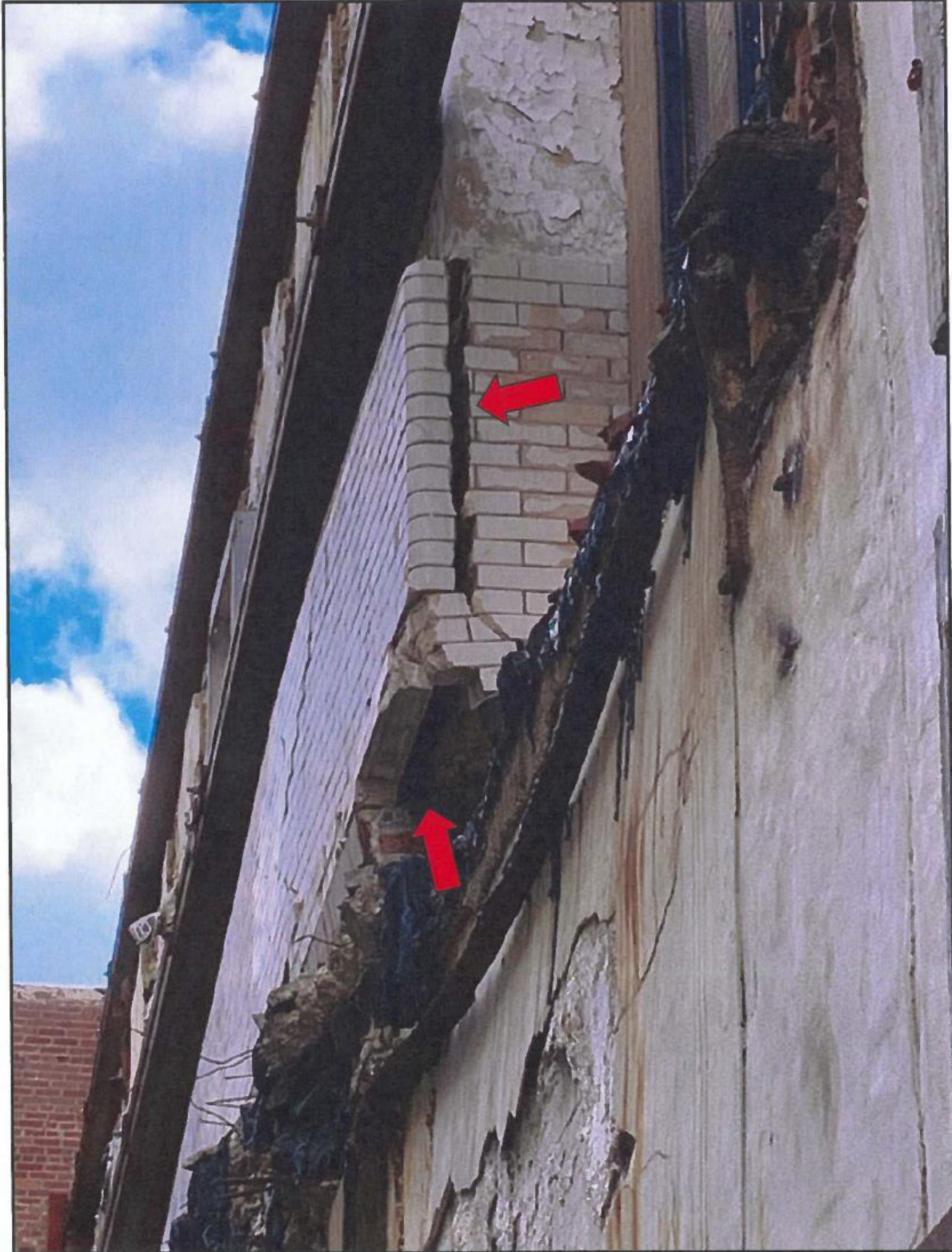
Image 24: Existing Conditions, Hendler Building, 2023
