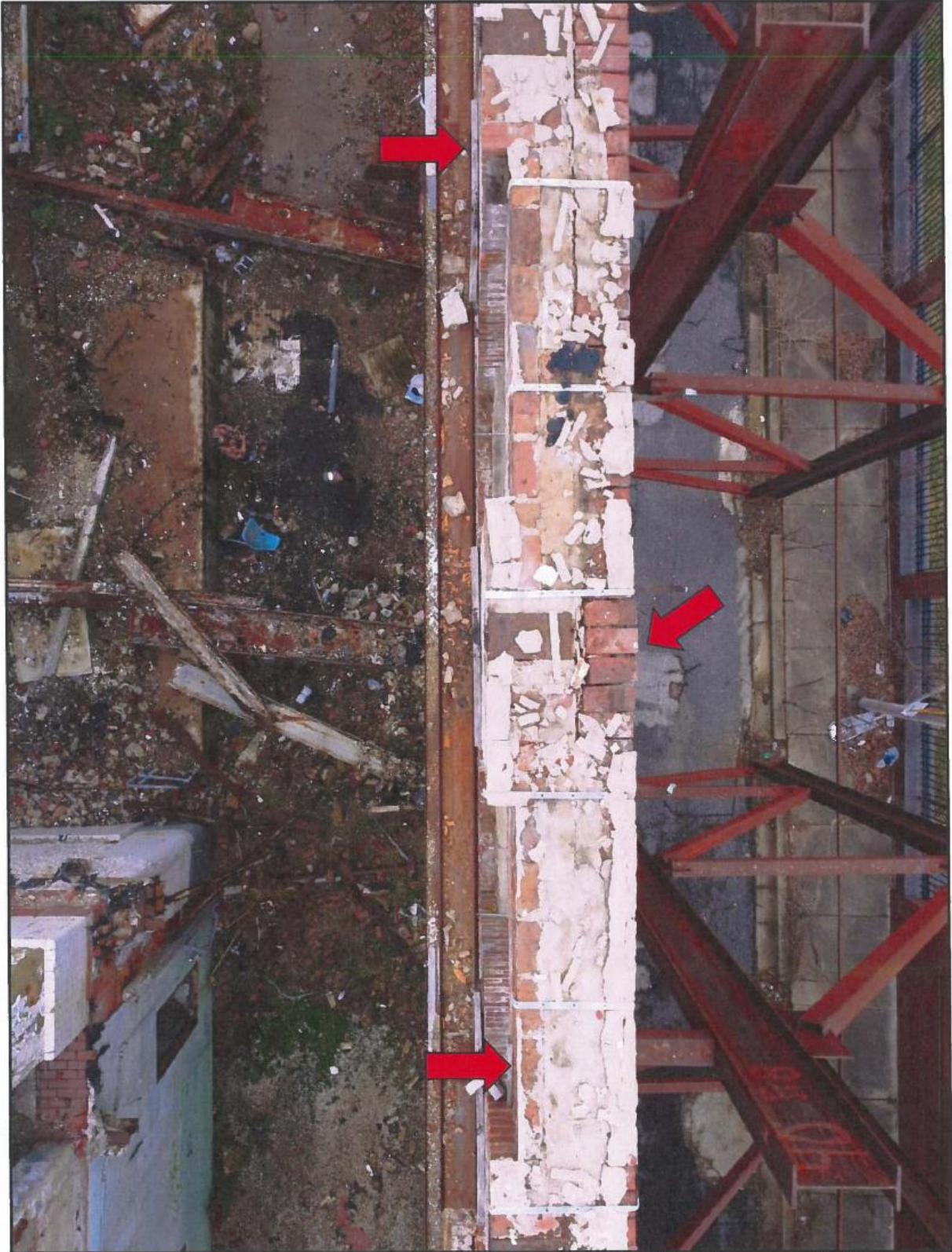
Image 27: Existing Conditions, Hendler Building, 2023
