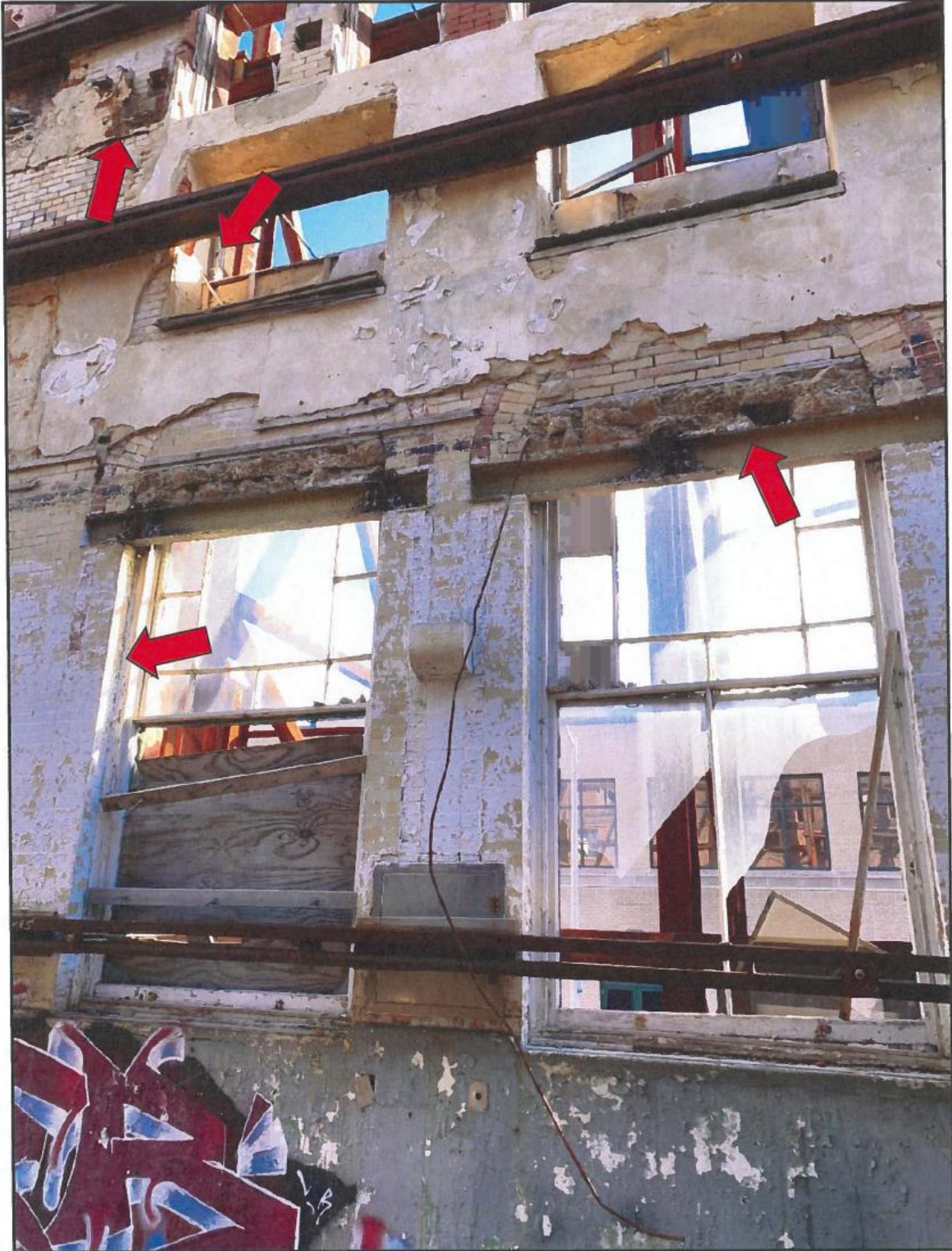
Image 17: Existing Conditions, Hendler Building, 2023
