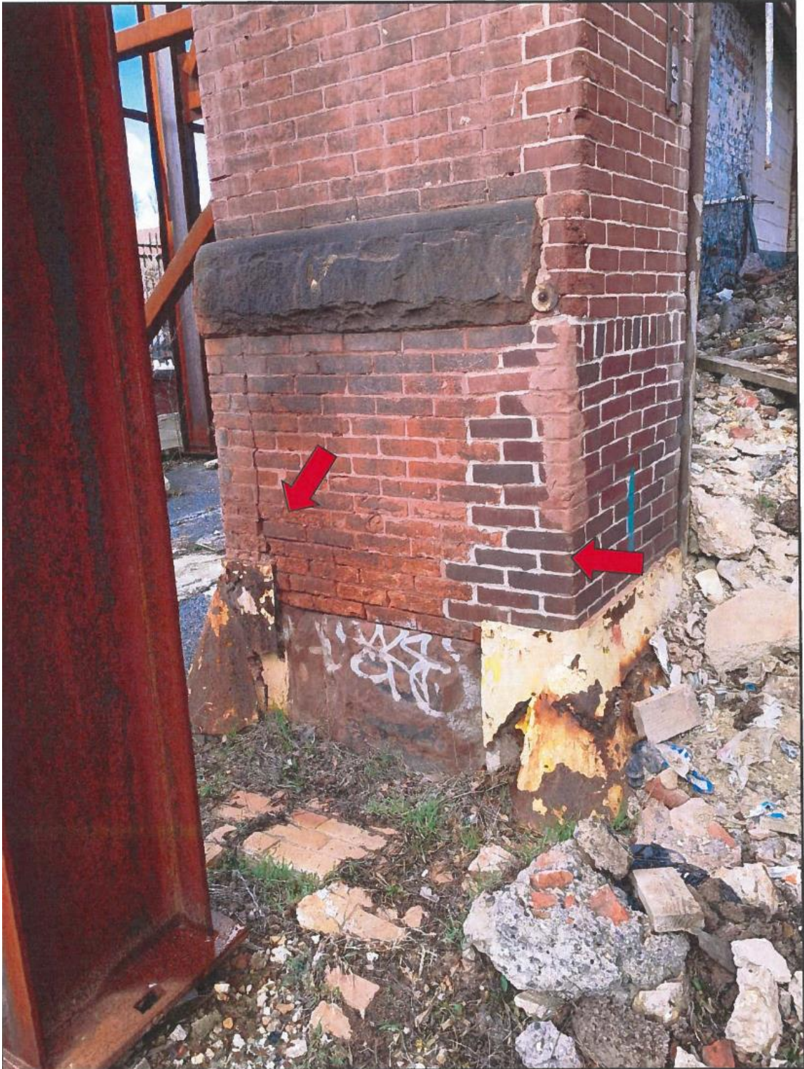
Image 14 Existing Conditions, Hendler Building, 2023
