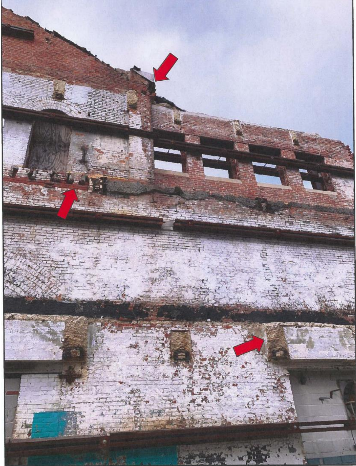
Image 34: Existing Conditions, Hendler Building, 2023
