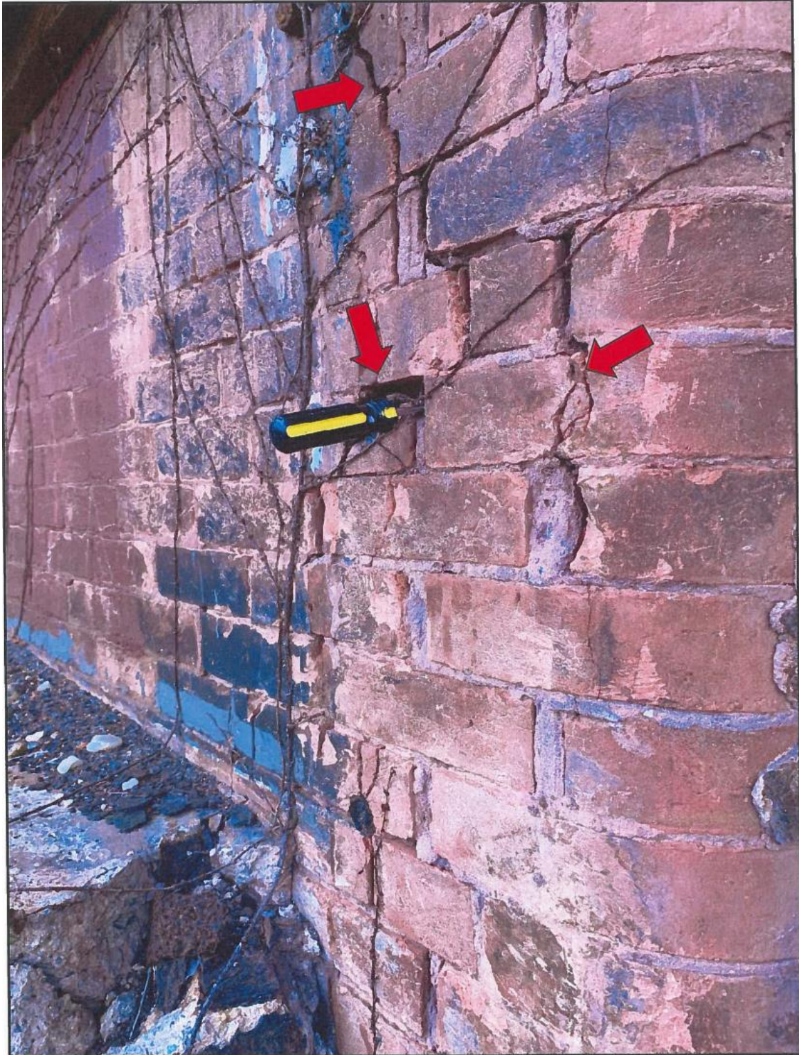
Image 31: Existing Conditions, Hendler Building, 2023
