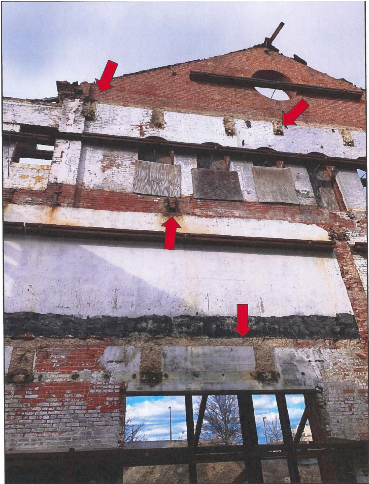
Image 33: Existing Conditions, Hendler Building, 2023
