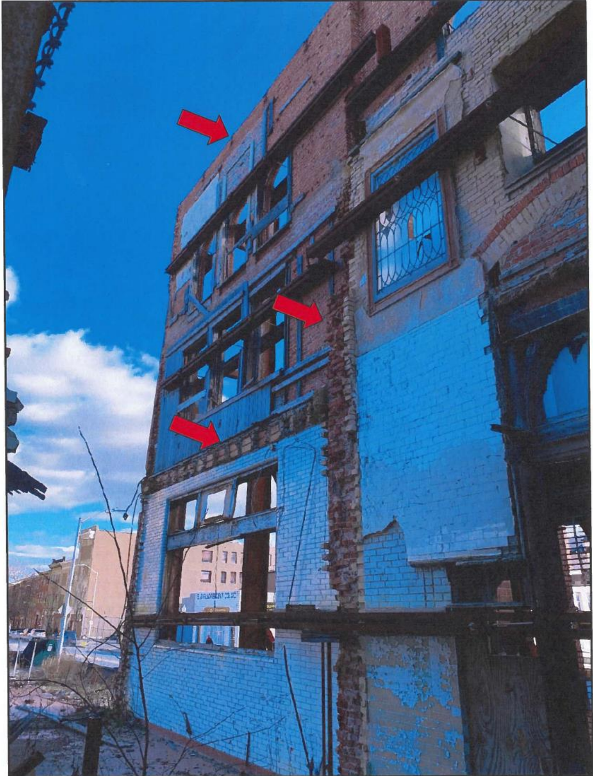
Image 16: Existing Conditions, Hendler Building, 2023
