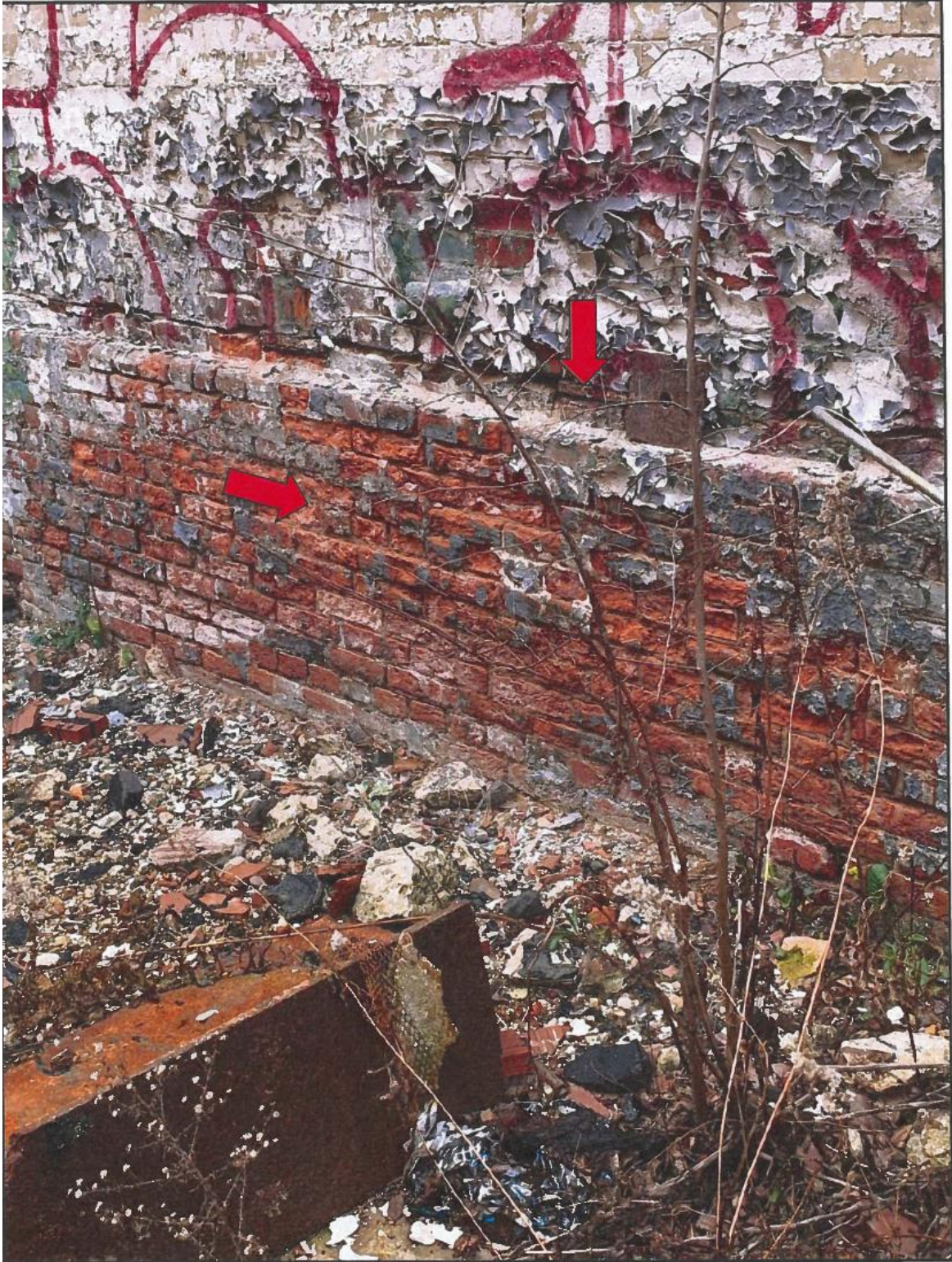
Image 25: Existing Conditions, Hendler Building, 2023
