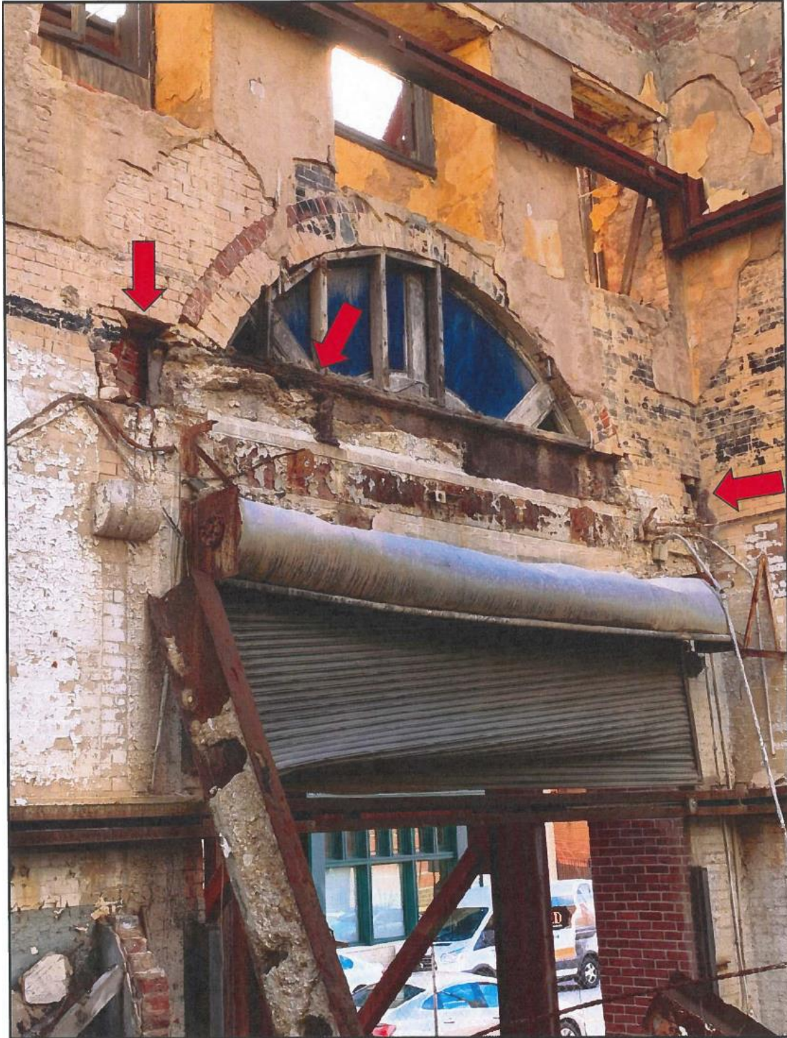
Image 18: Existing Conditions, Hendler Building, 2023
