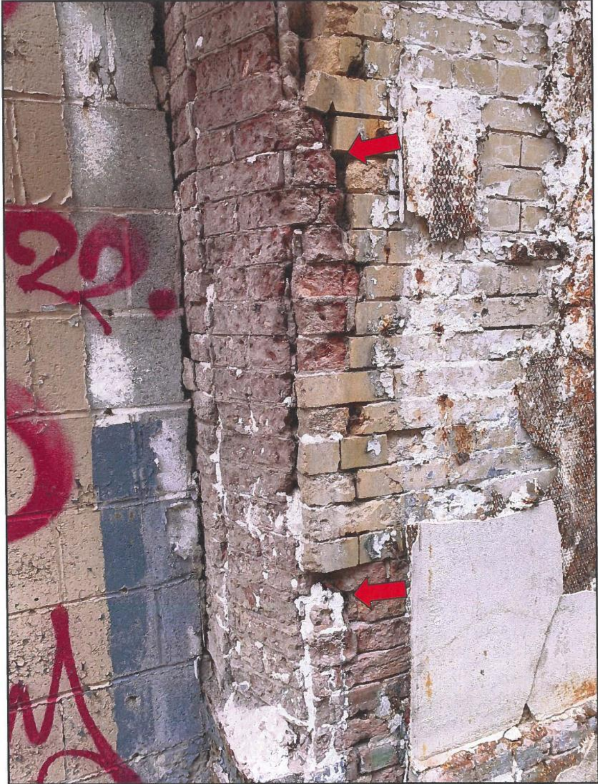
Image 26: Existing Conditions, Hendler Building, 2023
