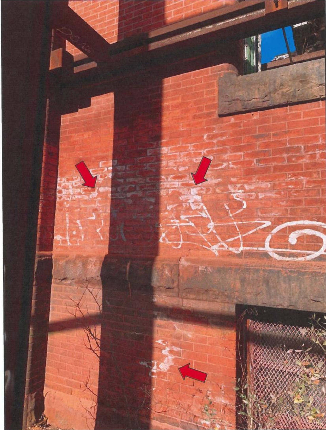
Image 12: Existing Conditions, Hendler Building, 2023
